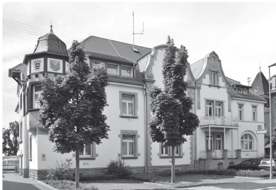
Police Headquarters Ladenburg in August 2010
