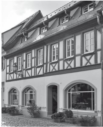
Building at Kirchenstr. No. 23 in August 2010
